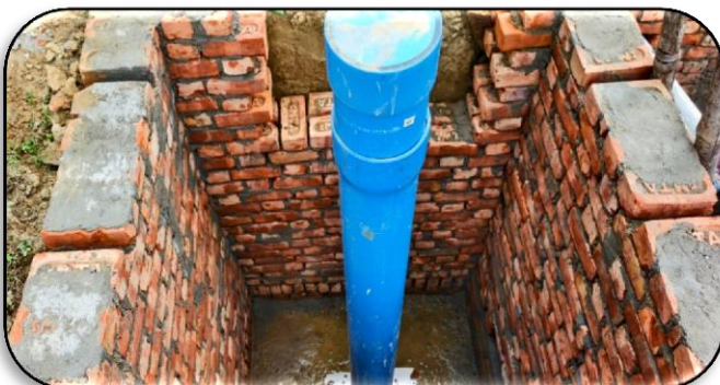
RAIN WATER HARVESTING (UNDER CONSTRUCTION)
